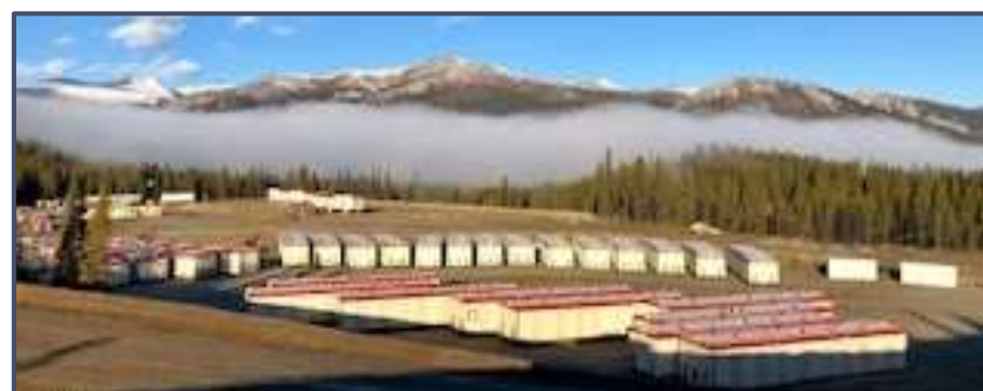
New camp facility
